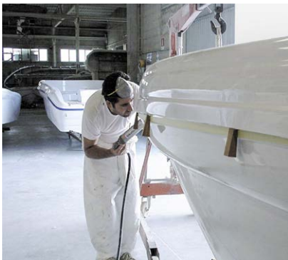
Fig. 8 Sealing with Sikaflex®-295 UV
