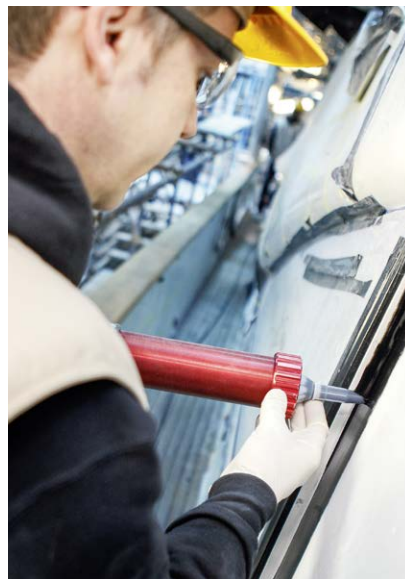
Fig. 6 Adhesive is applied to the window frame
