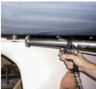
Fig. 12 The adhesive is applied
