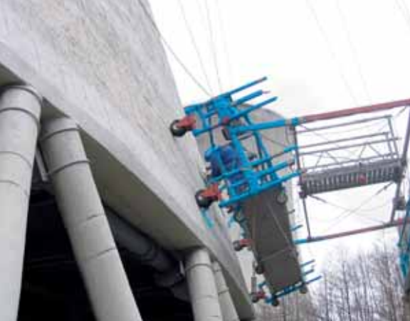
Concrete Coring in action
