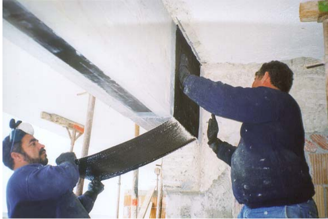
Fig. 9.5 Shear and Flexural Strengthening of a beam.
