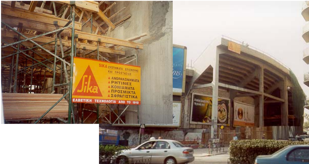
Fig. 9.3 Sport Stadium during Strengthening.
