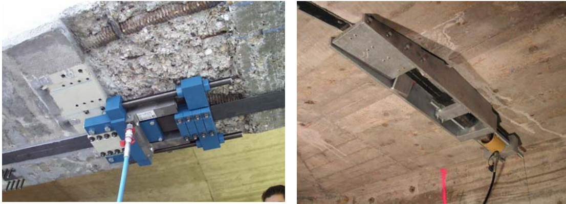
Fig 8.7 Sika Prestressed Systems; (a) Sika Leoba CarboDur II and (b) Sika-StressHead.
