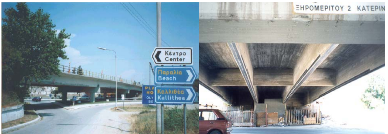
Fig. 9.2 Katerini Bridge and Strengthened Deck.
