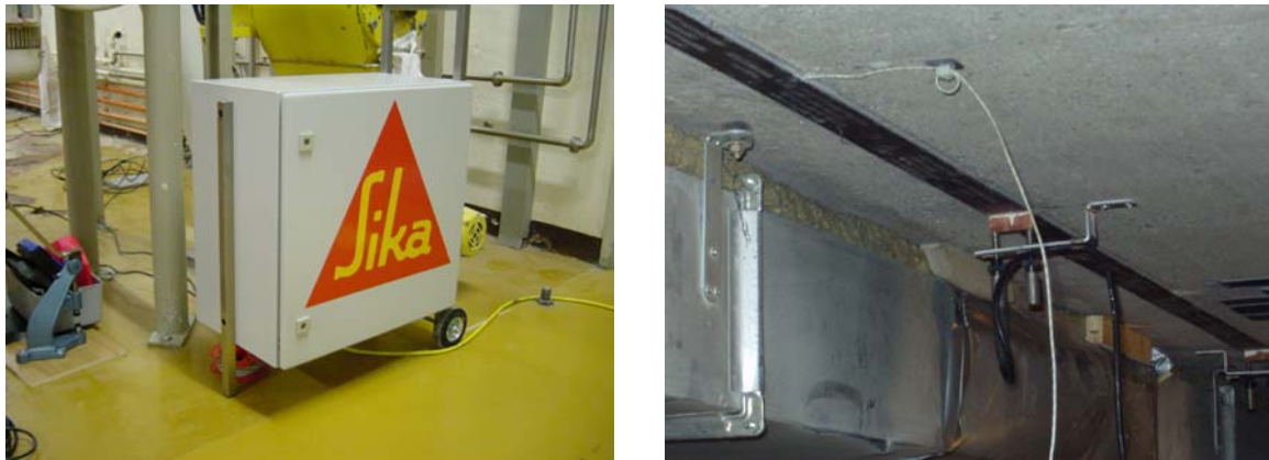
Fig 8.5 Fast Curing using Sika Heating Device.
