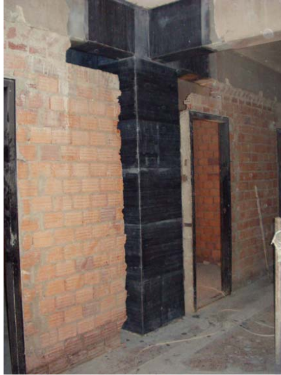
Fig. 9.11 SikaWrap Hex-230C Confinement of Columns and Joints.
