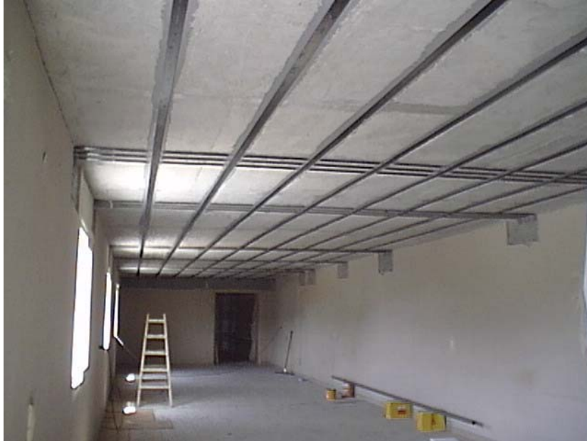
Fig. 9.7 Flexural Strengthening of a Slab.
