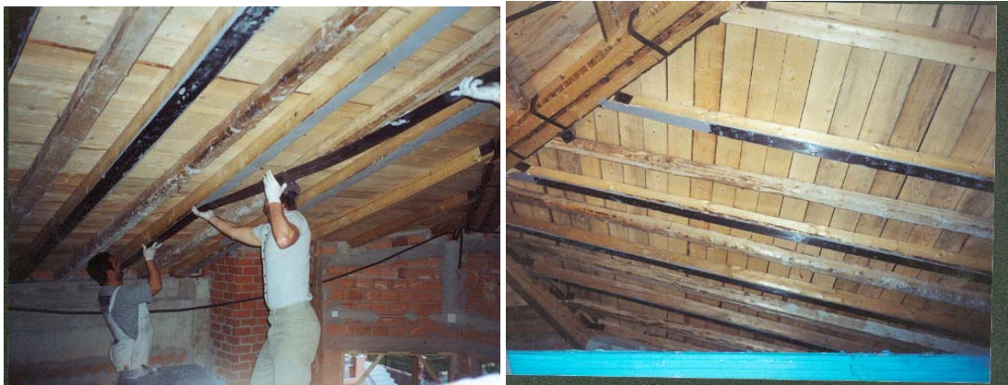
Fig. 9.6 Flexural Strengthening of a Wooden Roof.
