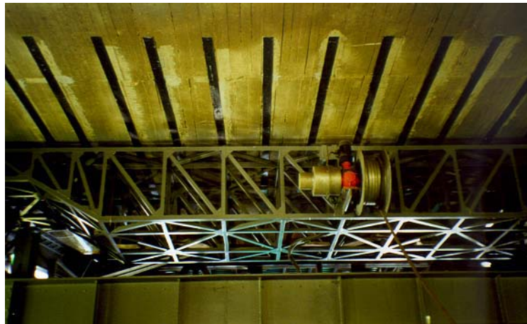
Fig. 9.1 Down side of Euripos Bridge Deck.
