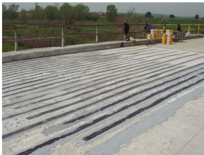
Fig. 9.8 Strengthening of Bridge Deck Slab over the Bridge Columns.
