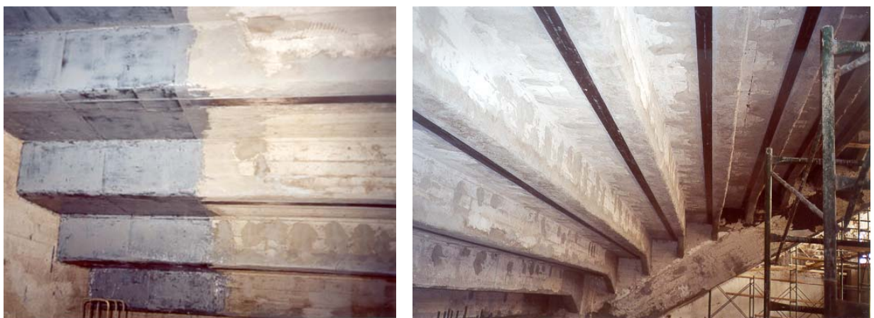
Fig. 9.4 Shear and Flexural Strengthening of Stadium Tiers.
