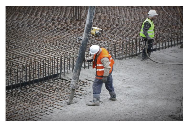
concrete mix which is impermeable to water. To achieve such quality, crystalline and pore blocker **Sika® WT-200 P** was used. **Sika® WT-200 P** consists of special active components which form non-soluble materials throughout the pore and capillary structure of the concrete and seal the concrete permanently against penetration of water.
