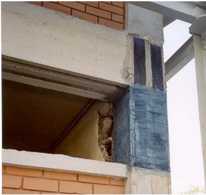
Fig. 5-3: Shear strengthening of: (a) beam end; (b) short column.
