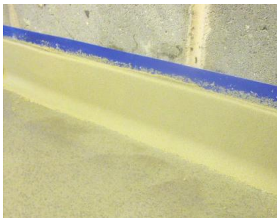
COVED SKIRTING APPLIED BEFORE FLOOR COVERING
